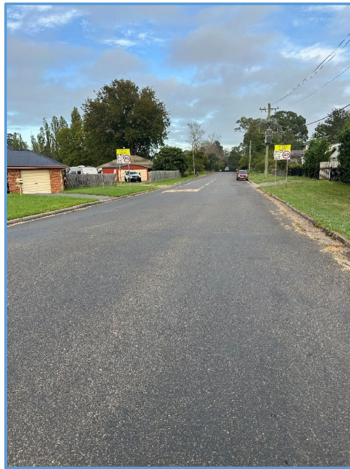
Figure 4c: Innes Road: Looking West from the intersection with Garrett Street
