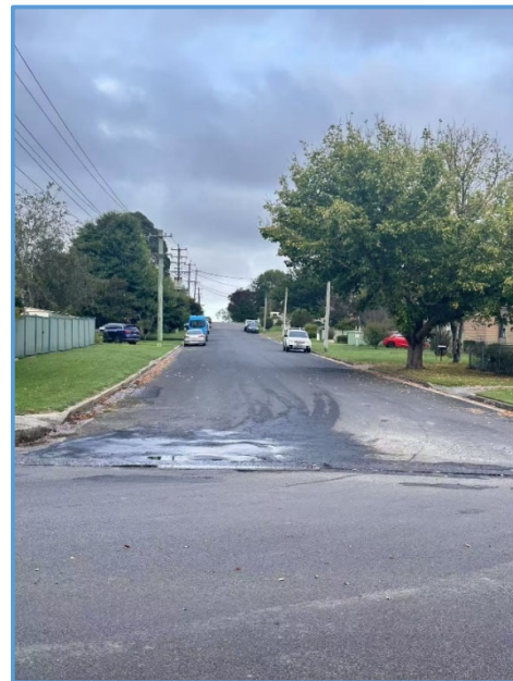
Figure 4b: Watson Road: Looking West from the intersection with Garrett Street
